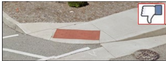
Detectable Warning Surface is not the full width of the ramp. See below for possible solutions.
